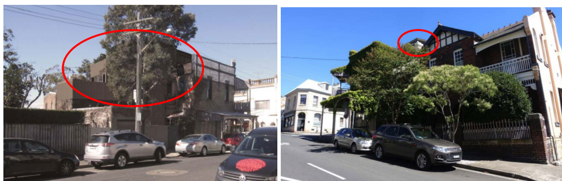
Figure 8: Views of proposal looking east (left) and north-west (right) towards 49 Darling Street Balmain East.
